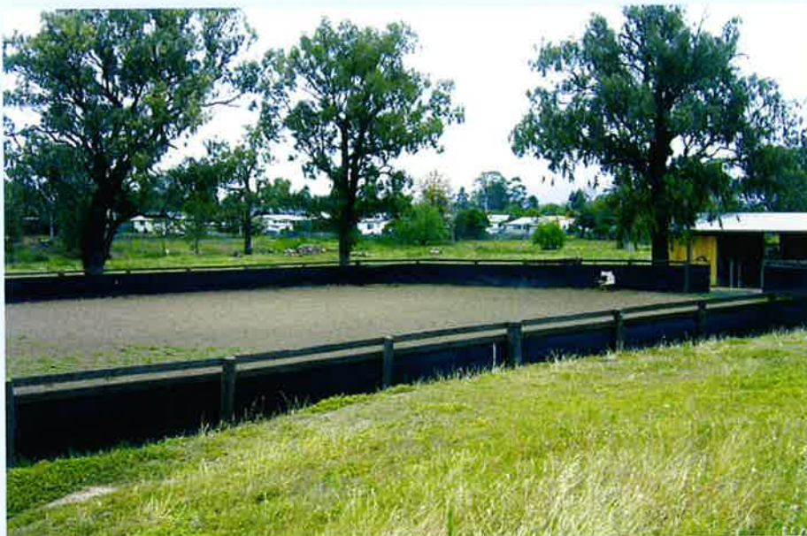
This is a typical horse yard installation using Splitbelt round the bottom to retain sand and provide a safer barrier. Hundreds of yards like this have been built using Splitbelt.
