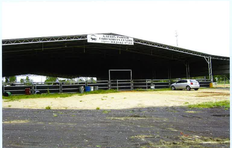
This indoor arena at Gatton, Qld has used Splitbelt extensively in its construction to provide safer conditions for the horses and riders. It is neat in appearance and is also easily fixed to either wood or steel structural members.
